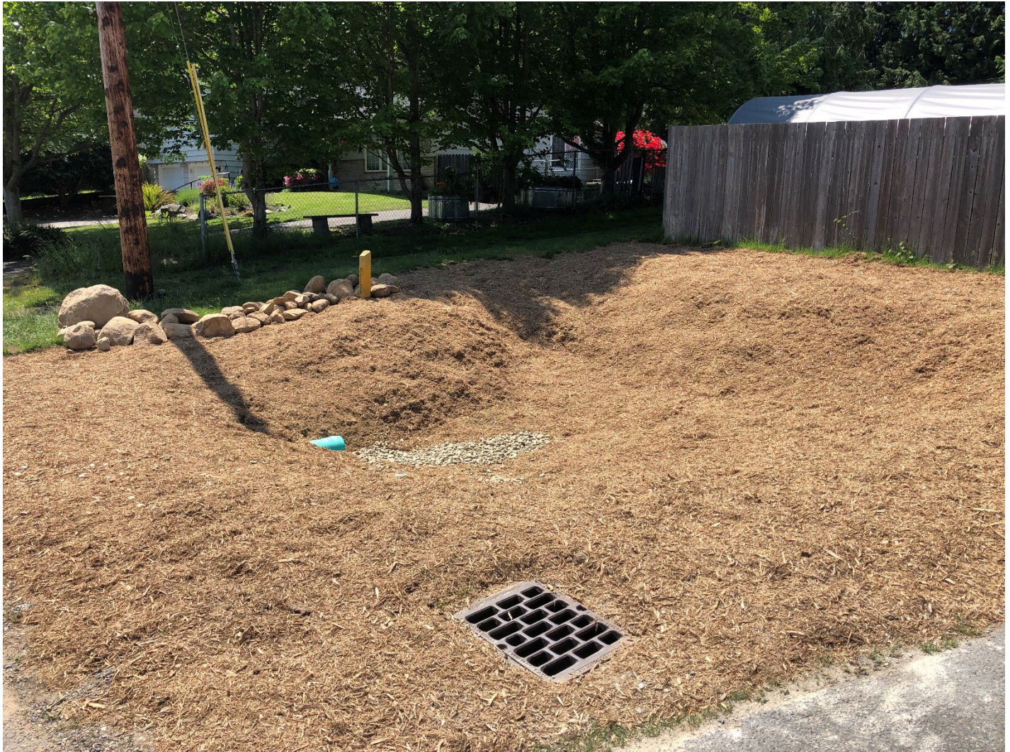
As the contractor, Snohomish Conservation District (SCD) excavated a large unused piece of land, where it was converted to a useful and beneficial rain garden. [Photo taken June 1, 2023]
